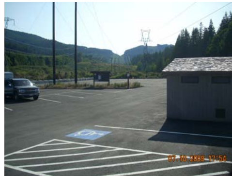
A view of the new Trailhead and CXT outhouse at Rock Candy Photo: DNR/Phil Wolff
